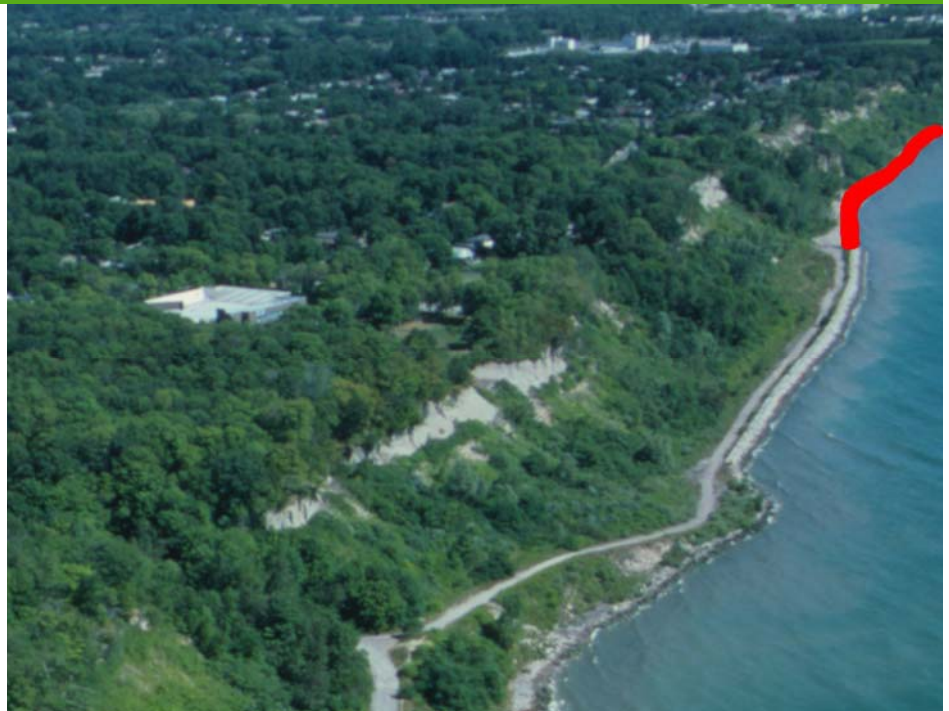
View of the shoreline below Guildwood Parkway, looking east from near the Guild Inn towards Morningside Avenue. Phase II of the project (highlighted in red) will stabilize another sector of shoreline to protect seven residential properties at the top of the bluffs.
